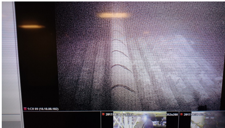
Crossing before Rock placement
